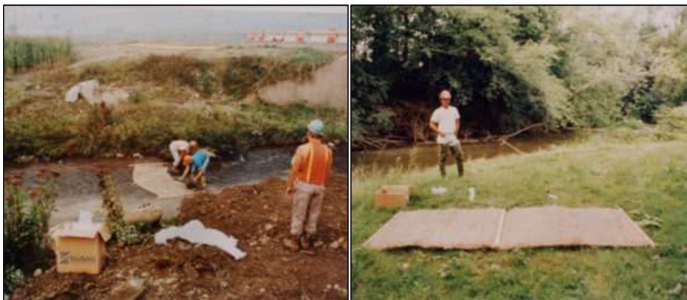
Plate 2-3 Typical Sedimat Details (Source: https://www.hy-tex.co.uk/ )
