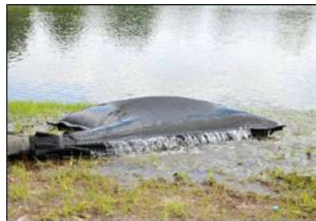
Plate 2-2 Silt Bag with water being pumped through
