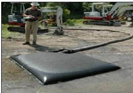
Plate 2-1 Silt Bag under inspection
