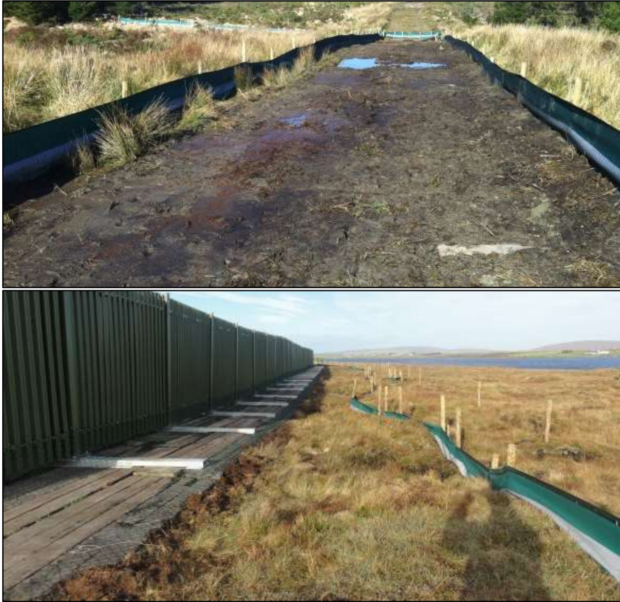
Plate 2-4 Typical Silt Fence Details
